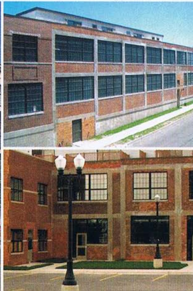
PHOTOS COURTESY OF RESEARCH LOFTS
